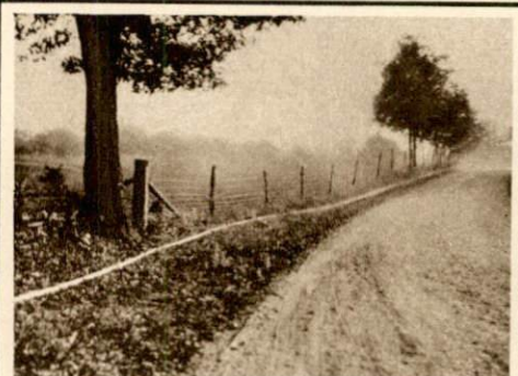
Oil pipe line (Stoll Oil Company), Legrande field.
