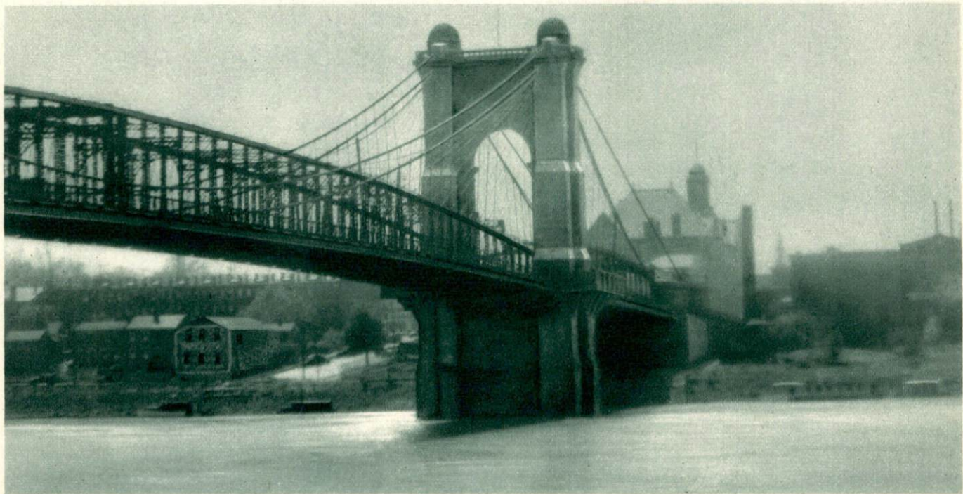
Covington end of suspension bridge.
