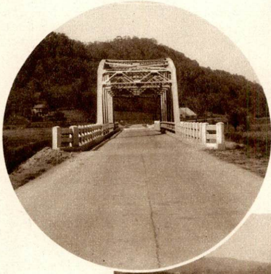
Below: One of the bridges.
