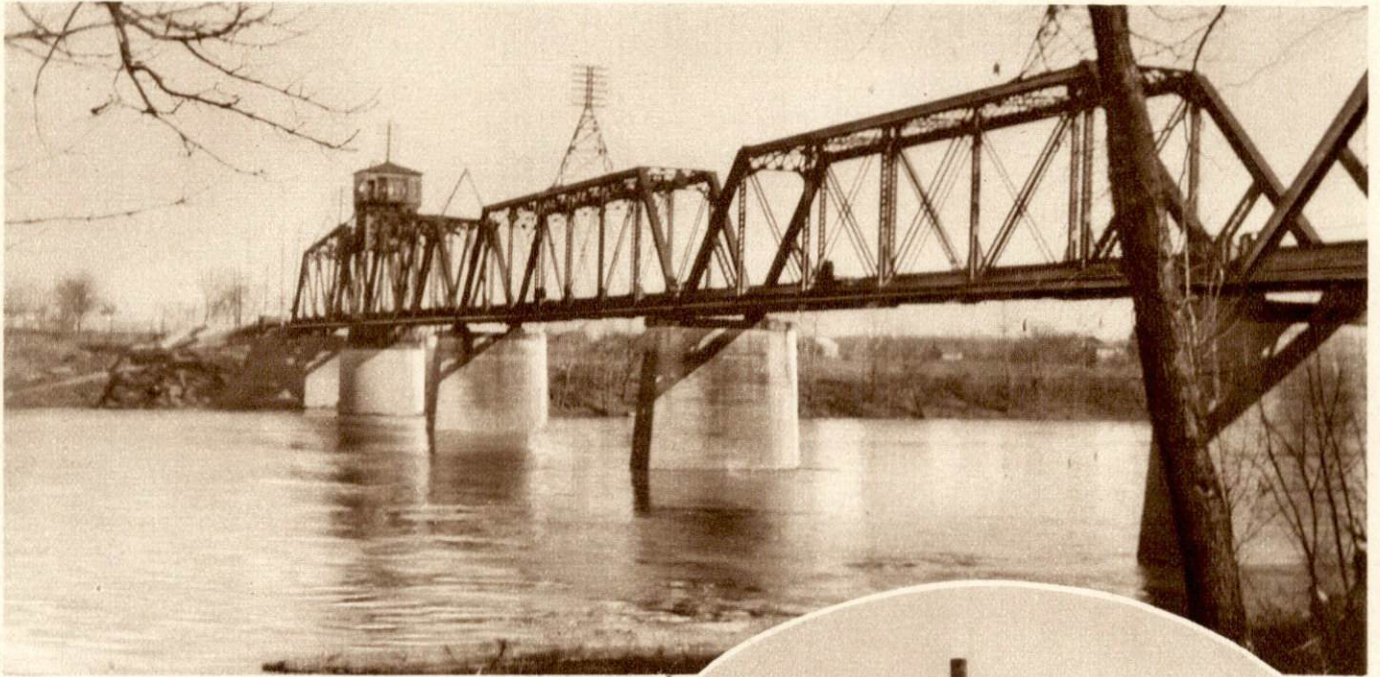
Illinois Central R. R. bridge across Cumberland River at Grand Rivers.
