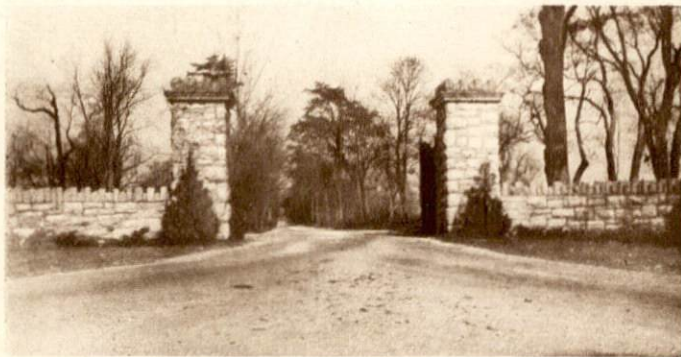
Entrance to Castleton Farm.
