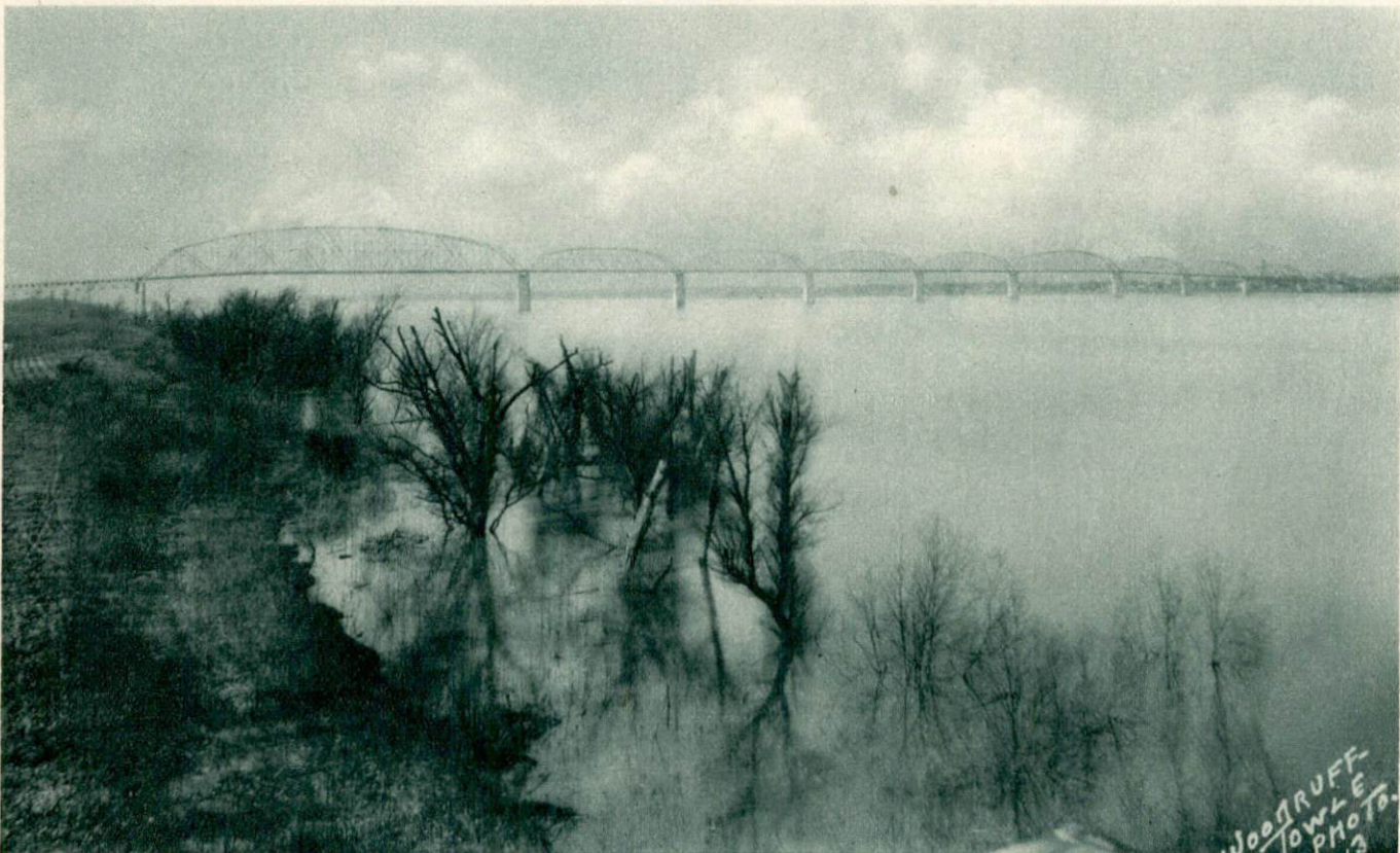
Paducah-Brookport bridge spanning the Ohio River at Paducah.
