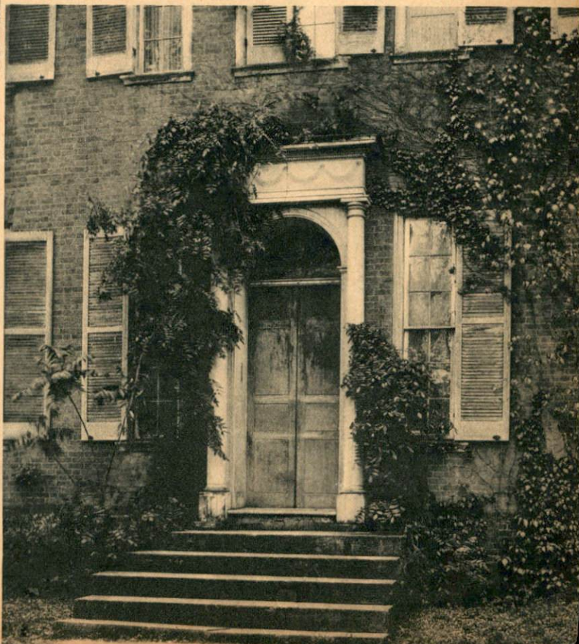
Below: The doorway, before its restoration
