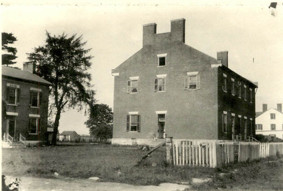
One of the four images recently acquired by the museum, this photograph includes (left to right) the 1846 Ministry Shop, the Meeting House Privy, Unidentified Shed, 1818 Meeting House, and 1841 Trustee's Office. The photo was taken after the Shakers left in 1922 and before the Meeting House was torn down in 1926.
