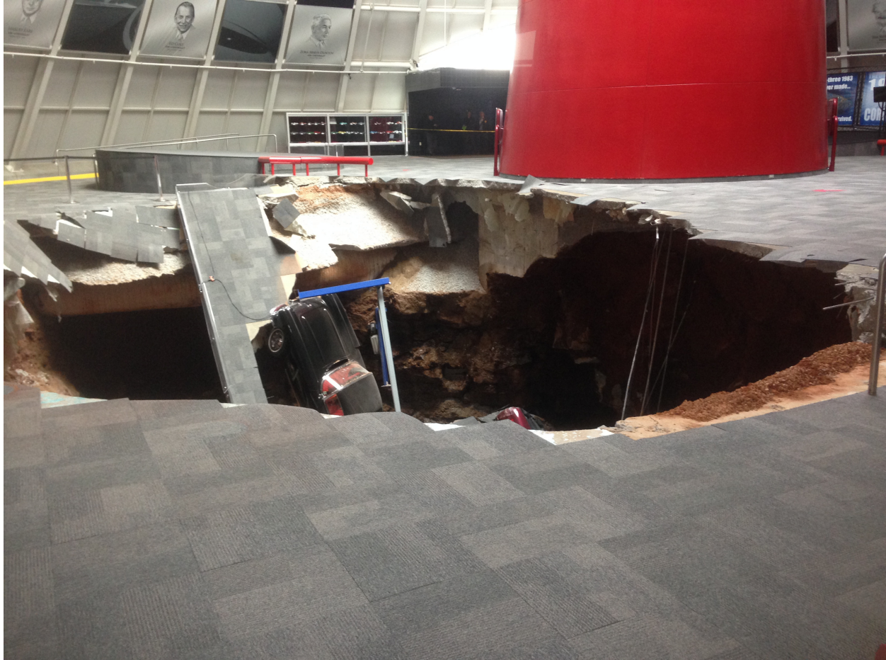
Figure 1. Initial sinkhole collapse: The original collapse on the day it occurred at the National Corvette Museum in Bowling Green, Kentucky.
