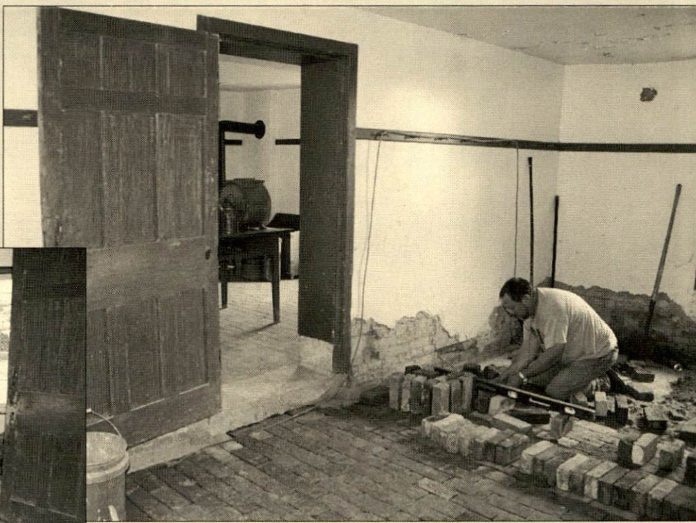
Contractor Johnny Miller supervises the restoration of the new brick floor in the dairy room. At left is the brick trough or sink used to help keep milk and butter cool. For more information about the restoration of the Smoke and Milk House, check out www.shakermuseum.com .
