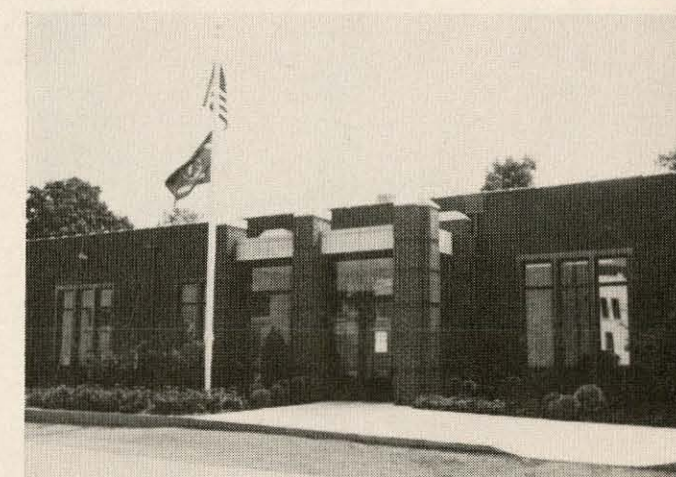
City Hall Annex
