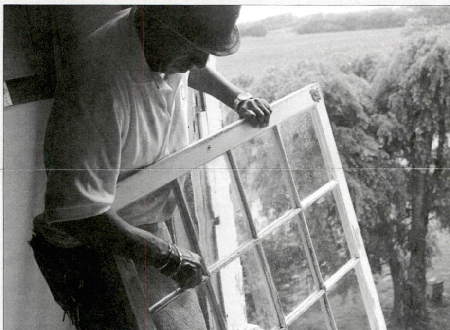
South Union Shaker Village restoration supervisor James Grinter works to remove failed restoration windows from the 1970s and to replace them with newly constructed replicas of the originals, thanks to funding from the Carpenter Foundation.
