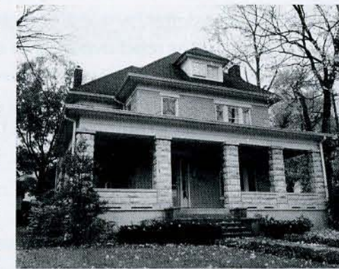
The Graham House at 1262 Chestnut is currently owned by Mike and Patty Minter. It is believed to be the only house in Bowling Green constructed entirely of concrete blocks.
