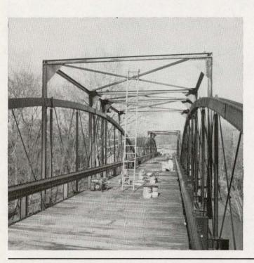
Restoration work is nearing completion on the Old Richardsville Road Bridge. David Garvin spearheaded the effort to repair this 100 year old bridge spanning the Barren River. This National Register structure is a triple Bowstring Arch Truss highly unusual in Kentucky.
