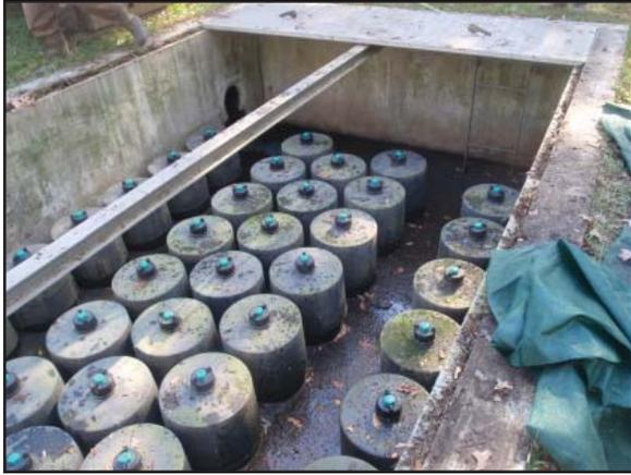
**Figure 1:** ZPG cartridges in filter system.
