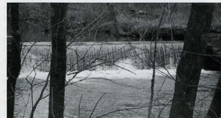
The old Dishman Mill dam on Jennings Creek.
