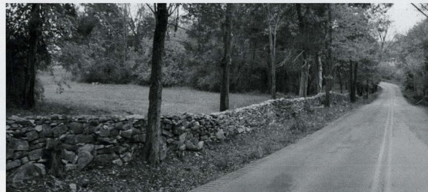
The stone fence bordering the Ennis property along Glen Lily Road. All photographs used for this story courtesy of Jeffrey Adams
