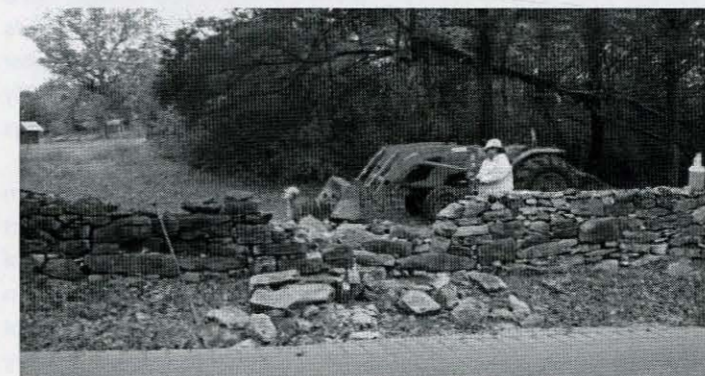
Repair work on the fence conducted by the Bricenos.
