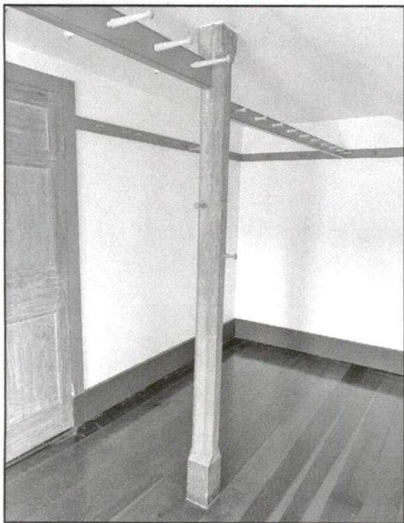
In the north "clothes room," suspended rails for pegs have been replicated using existing examples as patterns. These pegrails have been missing since 1935 when a bathroom was installed in this space.
