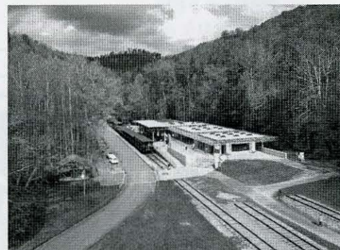
ABOVE: The terminus of the Big South Fork railway at the Blue Heron Mining Camp. After eating lunch, the group explored the nearby coal tippie, the entrance to the Blue Heron mine, and hiked around the area visiting interpretive sites and enjoying the fall foliage.
