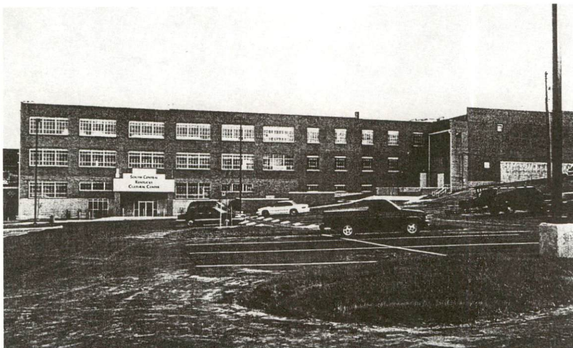
Main entrance canopy and parking lot.
