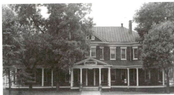
Front View of Baulch School
