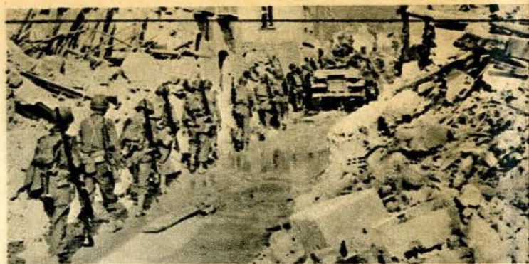
Reinforcements kept coming.
