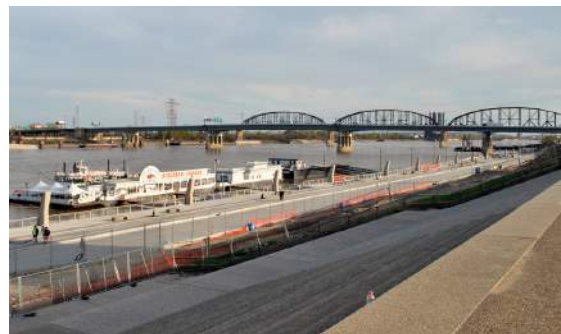
Figure 3.6: Poplar Street Bridge
