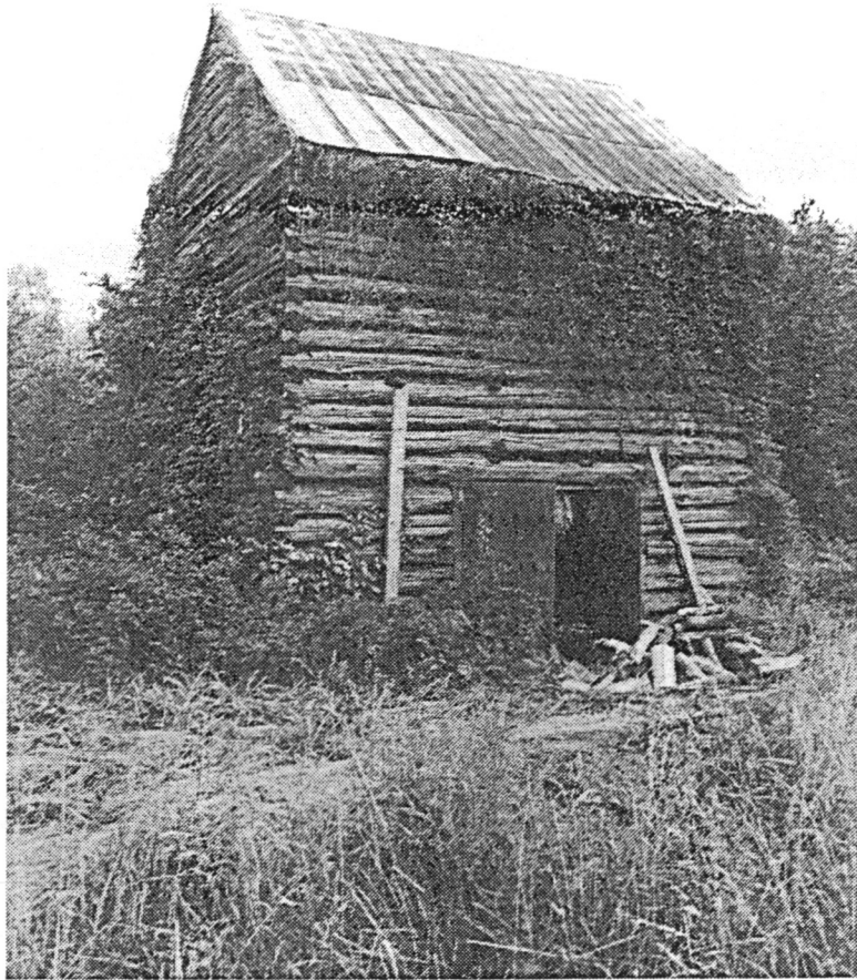
This older log dark tobacco barn, located near Redhouse, Virginia, is still used for the fire-curing process. Its form and dimensions are identical to many of the older log tobacco barns found in Calloway County, Kentucky.
