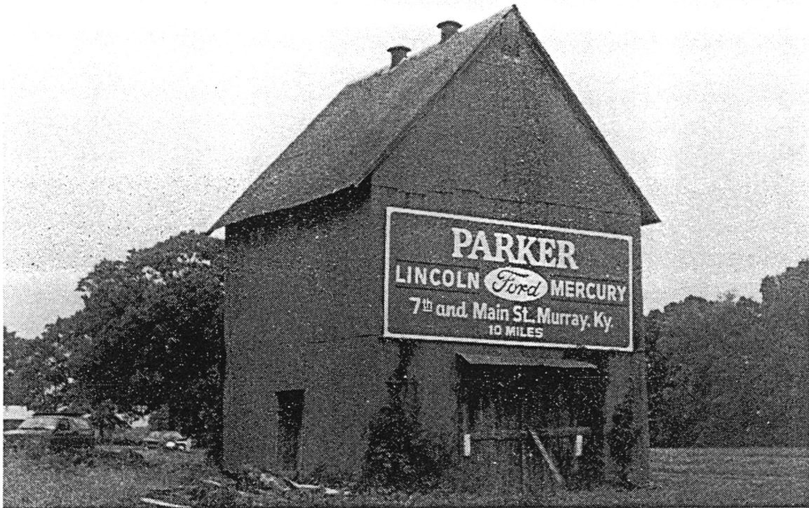
This fire-curing barn, located at the junction of Kentucky Highway 94 and Tidwell Road in Calloway County, measures twenty-four feet by twenty feet by thirty feet high. It is constructed of hewn logs and covered with corrugated tin. Note the original walk-through entrance on the side of the barn. The gable end double doors are a later renovation designed to accommodate tractor pulled wagons. This barn, too, was in use in the fall of 1992.
