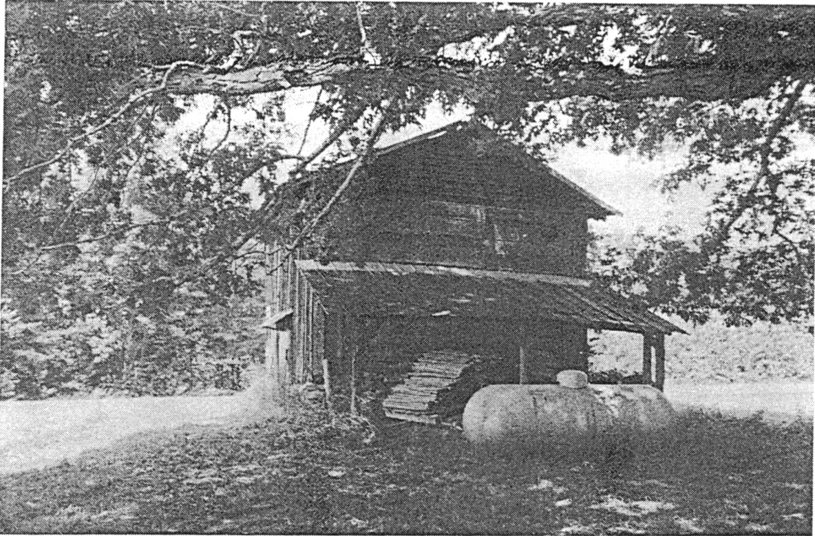
Many of the older flue-cure barns were converted from wood burners to kerosene, then to propane gas.
