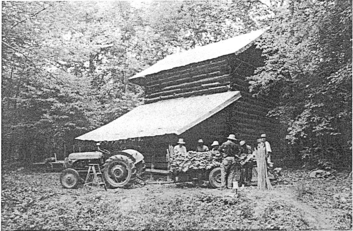
In past times, flue-cure tobacco was processed for curing just outside the barn in which it was to be loaded. The large shed additions to the flue-cure barns are for the protection from rain for those tending the fires. The sewing and staking of the tobacco could also take place under the shed in the event of inclement weather. This is the Page barn situated just south of Yanceyville, North Carolina.
