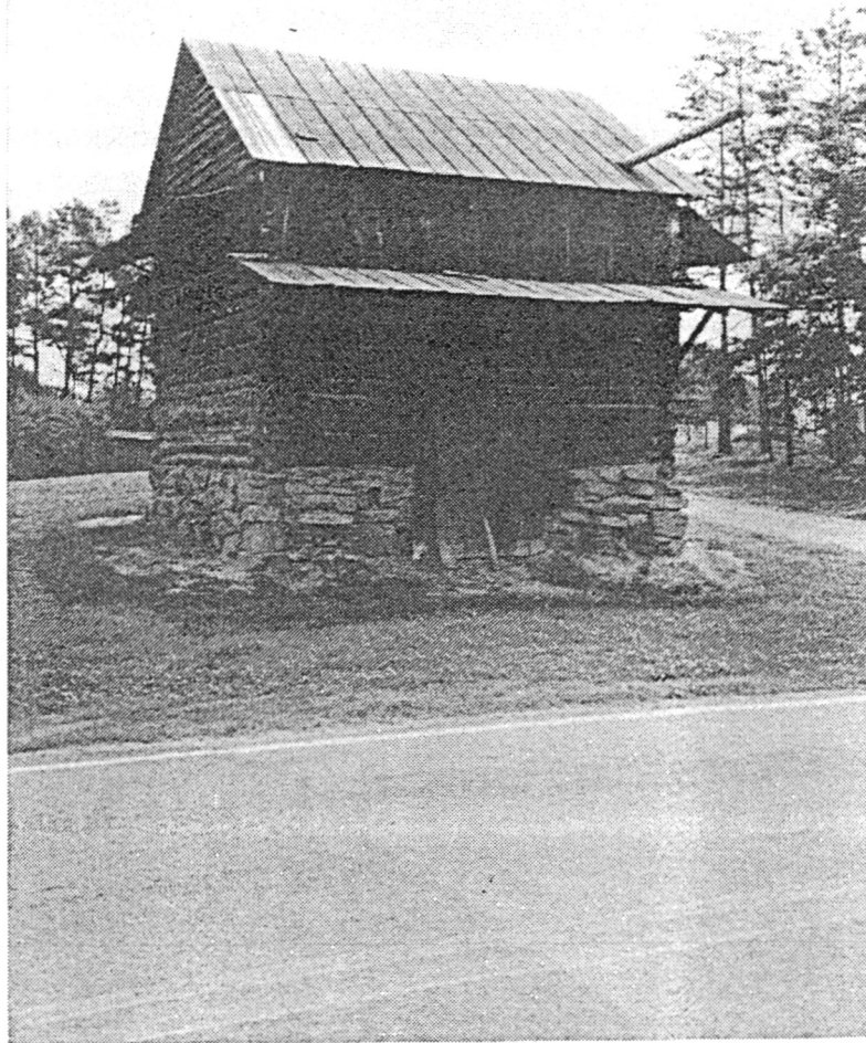
This log flue-cure barn is built up on a stone foundation which includes two externally fed furnaces. Note the pents or "bonnets" added to the gable ends to protect the logs from rain. This barn is located in Rockingham County, North Carolina.
