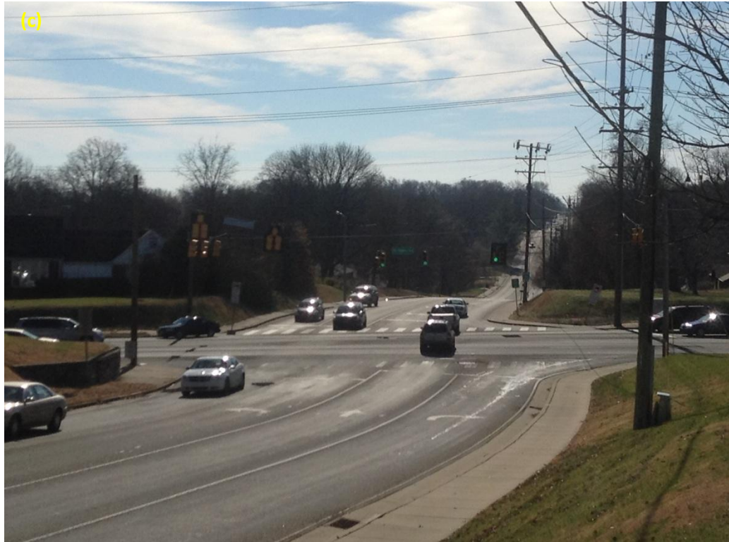
Figure 5.26. Photo Taken at Point c near Nighttime Hotspot 8.
