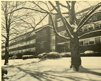
Thompson Complex was one of ten buildings that received major damage over Christmas.
