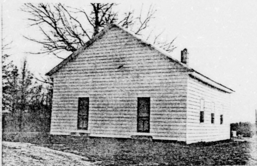
Fig. 1.--Exterior view of Oak Forest Baptist Church. A log building that has been covered with a siding. (near Richardsville, Kentucky).
