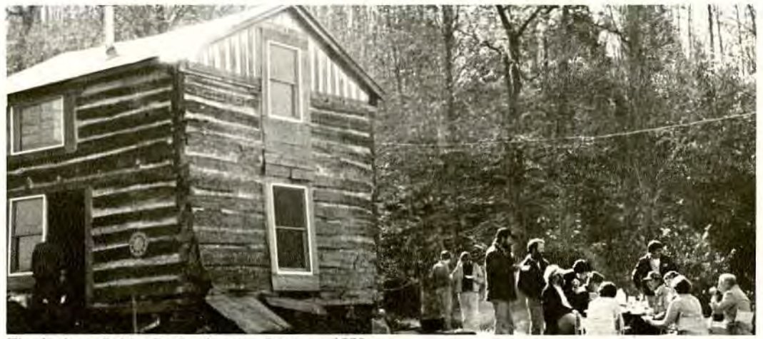
The Jackson Cabin, Butler County, October, 1979.
