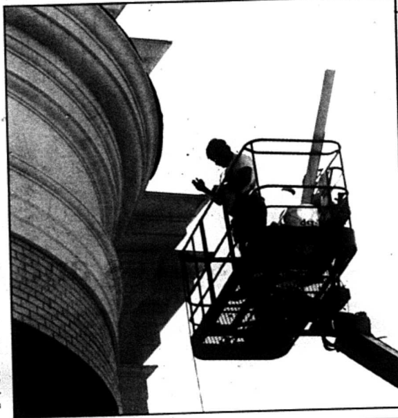
Merrick Construction employee Ralph Arnold of Louisville covers soffit ledges with metal at the First Baptist Church construction site on Monday. The church, which is being rebuilt after fire destroyed the sanctuary in 1991, is scheduled to hold its first service in the new sanctuary on Nov. 13, according to Pastor Richard Bridges.
