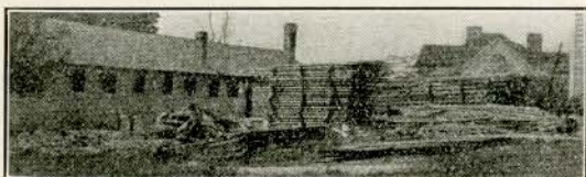
The old barracks have been torn down. They occupied the site of the new Training School Building.
