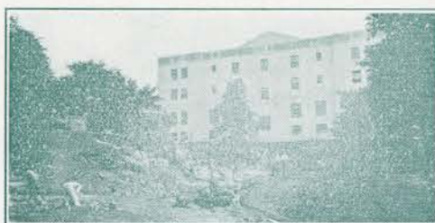
Excavating for Swimming Pool Adjoining Physical Education Building
